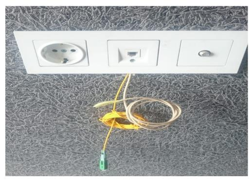
METHOD-1 Terminating the fiber coming out of the socket by mechanical connector.
